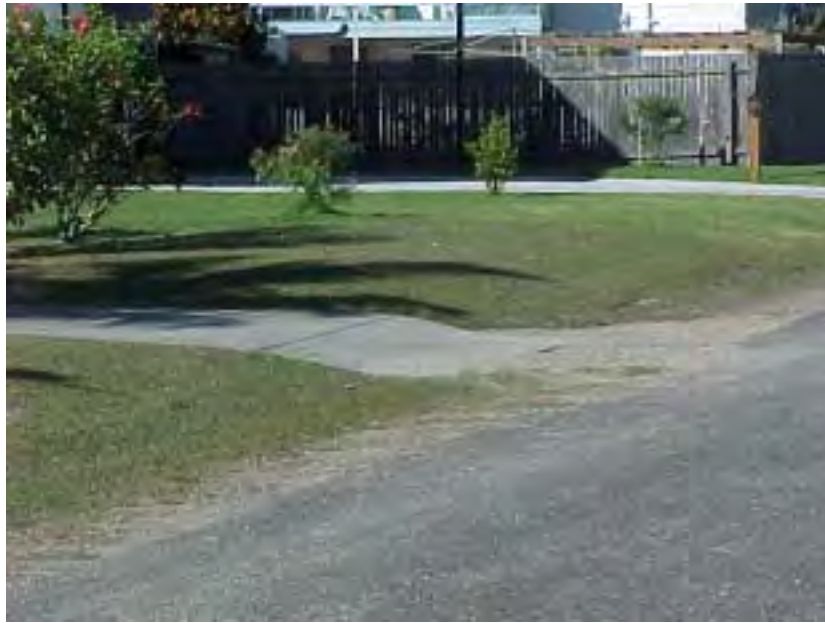
Figure 3.2 Typical roadside swale
